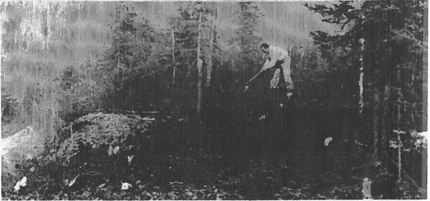
EAGLE RIVER CAMPGROUND during construction.
